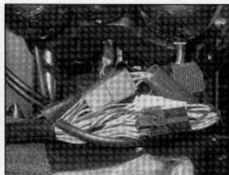
15.1b On early faired models, the connectors are housed inside a cover that sits on top of the headlight
